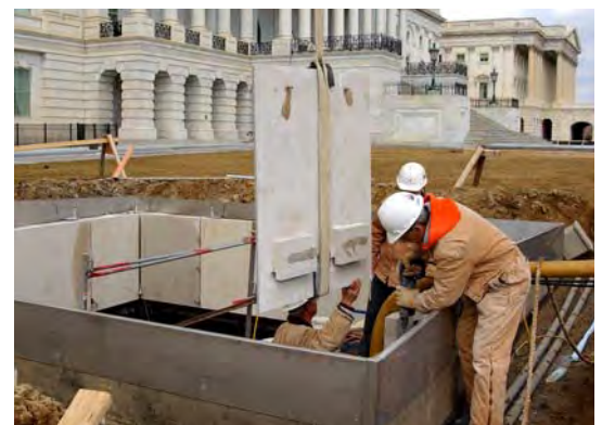
Stone masons install sandstone around a CVC skylight.
