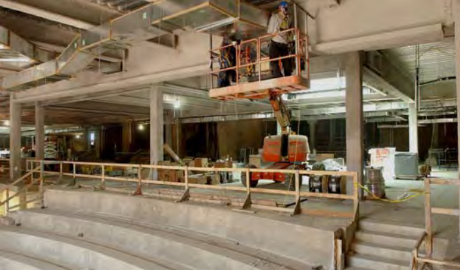
Workers install ductwork in a CVC orientation theater.
