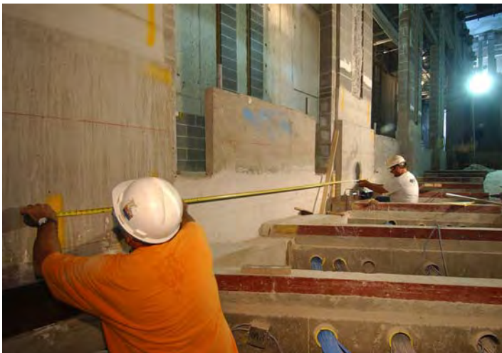
Stone masons establish guidelines for layout of stone in the Congressional Auditorium.
