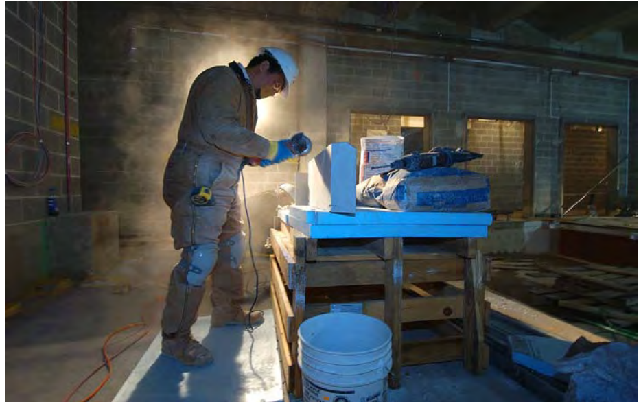
A stone mason trims a piece of sandstone at the north end of the Visitor Center Exhibition Hall.
