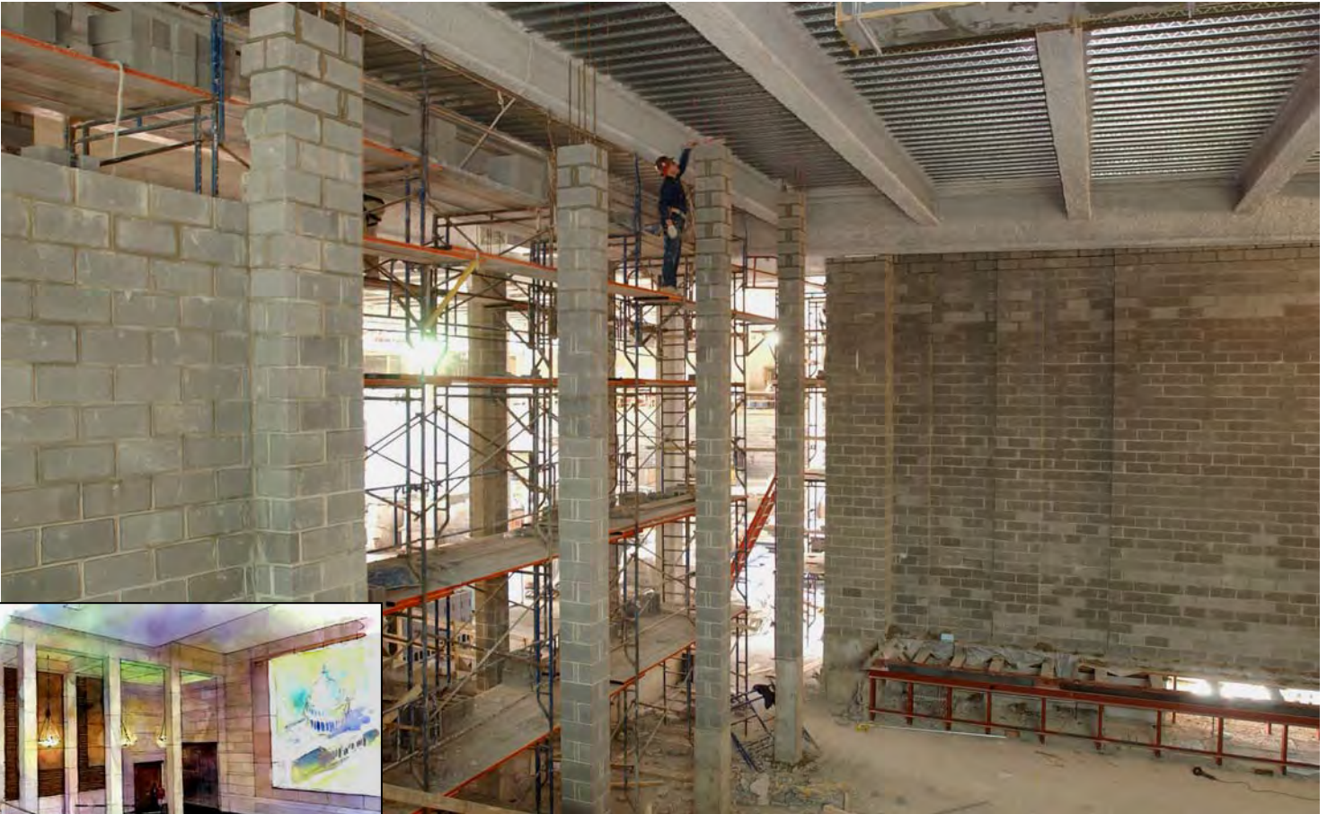
Above: A worker completes a blockwork column inside one of two CVC orientation theaters. Inset at left: An artists rendering of a completed orientation theater. A 12-minute film about the Capitol and the Congress is being produced and will be shown three times per hour in each theater.
