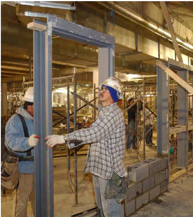
Above: Workers install one of several hundred door jams that are included in the CVC floor plans.
