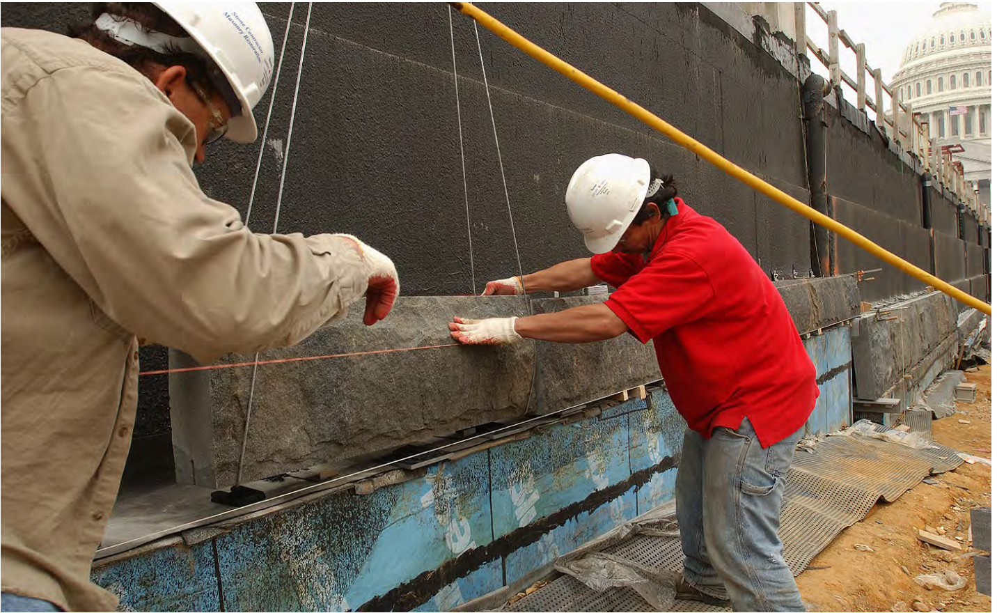
Stone masons set a granite block to the north exterior wall of the Congressional Auditorium. The rough cut of the stone echoes the historic perimeter walls.
