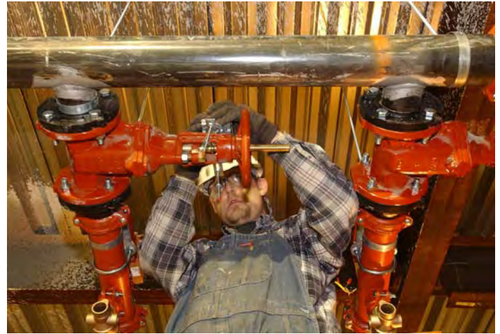
A sprinkler fitter installs a sprinkler system valve.
