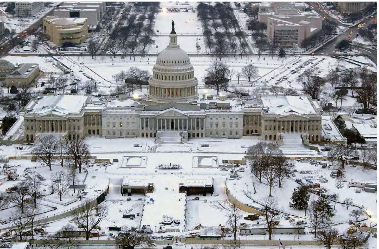
A view of the East Front Plaza as it appeared Wednesday, Jan. 19, 2005, the afternoon before the Presidential Inauguration. Crews worked diligently to remove tons of snow from both the East and West Fronts of the Capitol to clear the way for inaugural activities.
