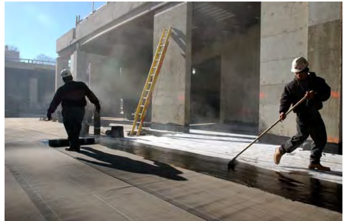
Workers place a waterproofing membrane at the CVC entrance zone.
