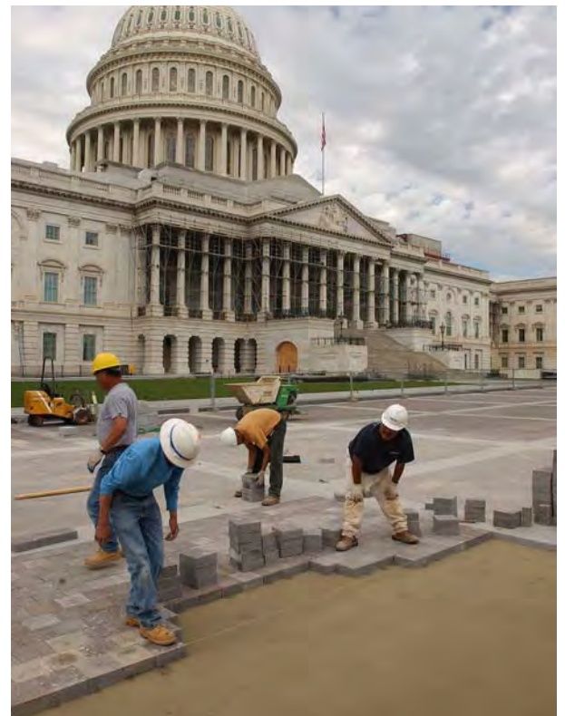
A crew installs granite pavers on the East Front Plaza.
