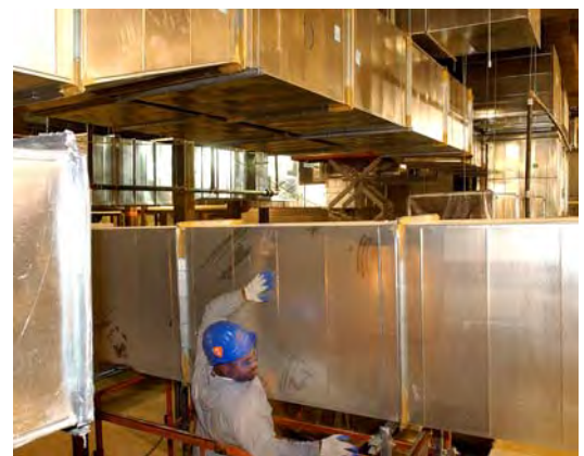
A worker installs air handling ductwork in the CVC.
