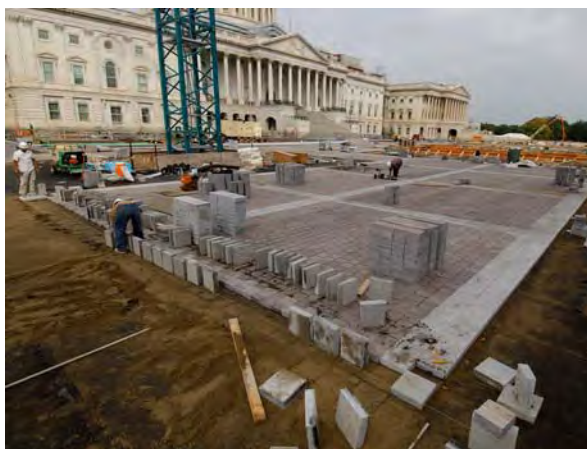
Below: Workers continue to place granite paving stones to prepare the western half of the East Front Plaza deck for the Inauguration in January 2005.
