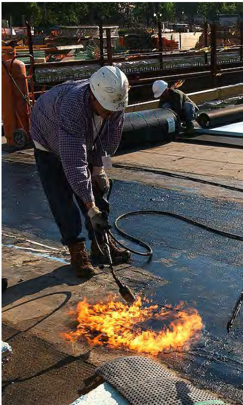
A blow-torch helps to seal a waterproofing membrane.
