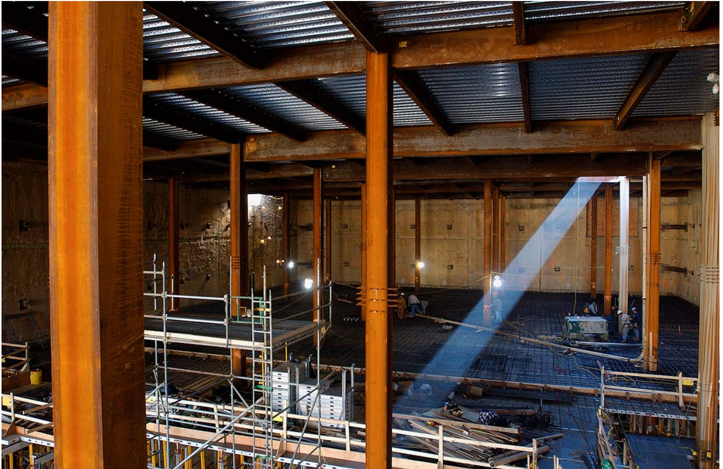
A beam of sunlight penetrates a temporary opening in the CVC roof deck in the southwest quadrant of the site where crews are busy assembling the formwork for the lower-level floor slab. Concrete placements for the floor slab are expected to occur this week.
