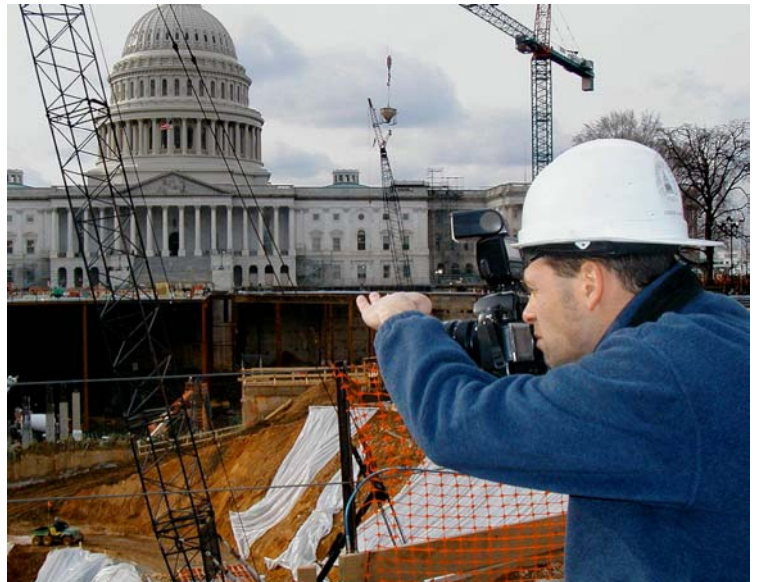
AOC photographer Chuck Badal has taken thousands of photographs of CVC construction activities since work began late in 2001. Chuck is responsible for the majority of photographs that have appeared in the CVC Weekly Construction Summary and on the CVC web site.
