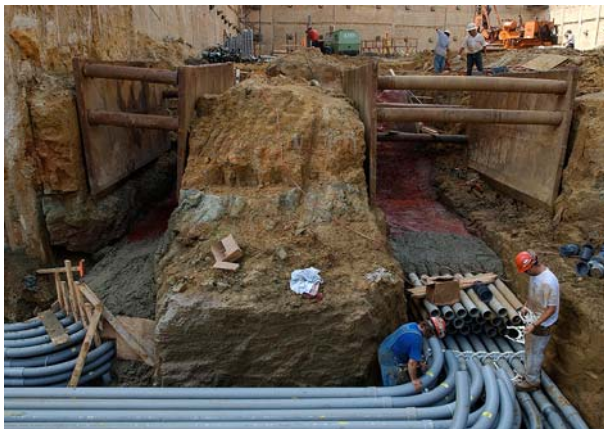
A 60-inch-diameter auger is used to excavate 15-foot-deep holes that will house concrete caissons. The caissons will serve as footings for 50-foot-high steel columns.
