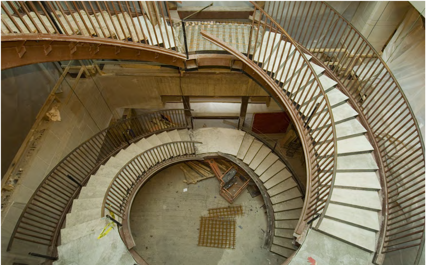
A spiral staircase winds down through all three floors of the Senate Expansion Space. The House Expansion Space features a similar staircase.
