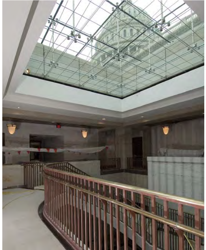
A skylight above the stairwell atrium in the Senate Expansion Space provides a dramatic view of the Capitol Dome. The staircase connects all three levels of the Senate Expansion Space.
