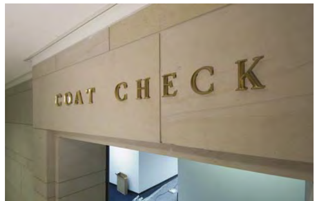
Bronze letters are now being installed in the CVC to identify interior spaces.
