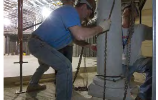
Masons install a sandstone column in a CVC Gift Shop.
