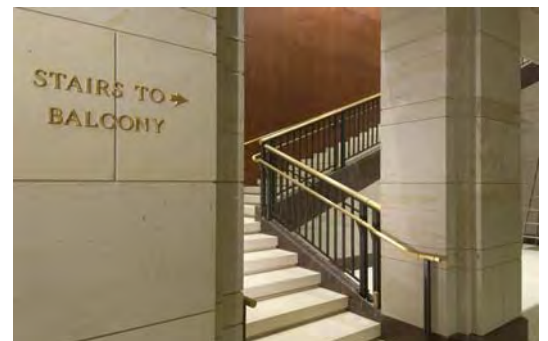
Bronze pin-mounted letters identify interior spaces and way-finding paths throughout the CVC.
