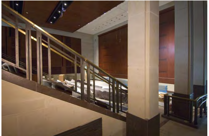
Bronze railings, millwork, and stone work are complete in the North Orientation Theater.
