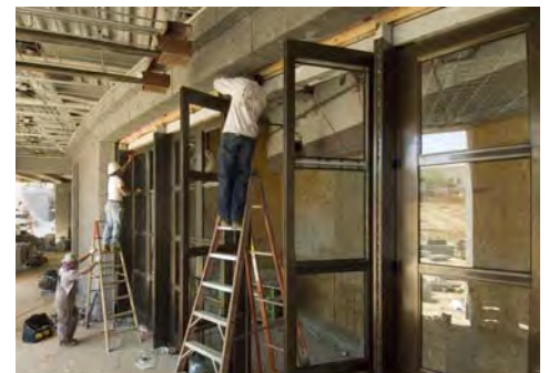
Workers install 12-foot-high bronze doors at the CVC's north entrance zone.
