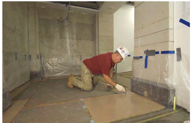
A worker applies an epoxy that binds the stones within a terrazzo floor. This corridor connects House-side elevators to House Expansion Space.
