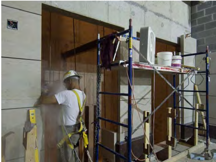
A stone mason sets stone around a new elevator opening.
