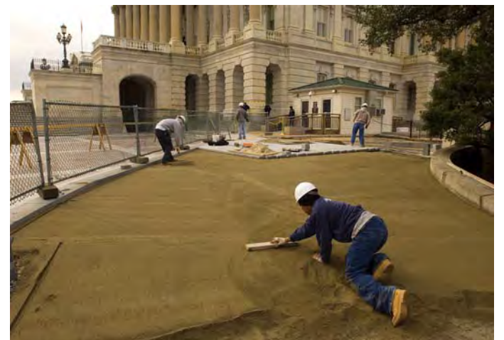
Clockwise from above: A welder connects water lines inside the CVC utility tunnel; Workers inside the Great Hall prepare to raise a sandstone block for one of the ceiling soffits between ceiling vaults; a worker installs a portion of the ceiling support structure in a corridor near the Great Hall; masons prepare a sand and cement bed for granite pavers for the sidewalk leading to the Senate Carriageway and North Door. Most of the stonework in this area will be complete to a level sufficient to support pedestrian and vehicular traffic for the State of the Union address on January 31, 2006.
