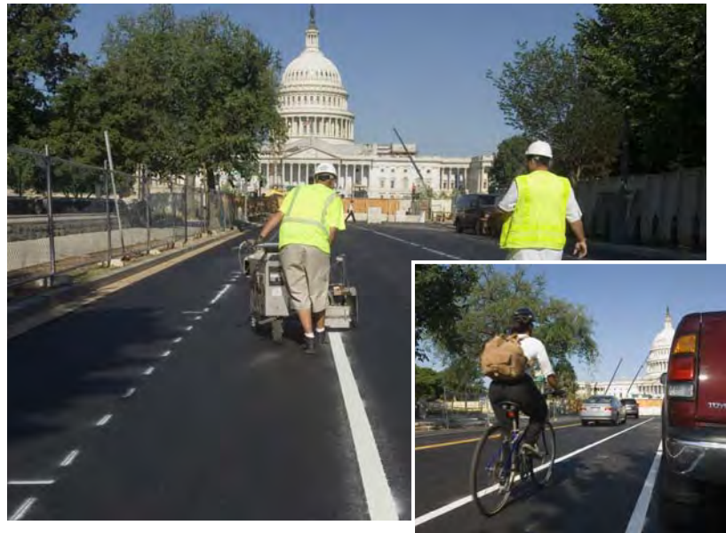
Above: Painters stripe the traffic pattern on East Capitol Street. Inset: A day later, on June 14, 2006, the street was open to vehicular, pedestrian and bicycle traffic.
