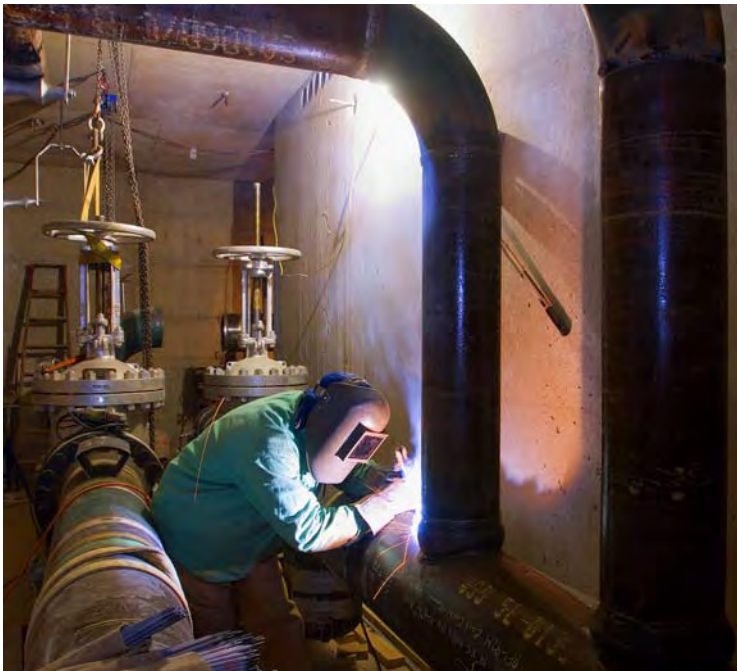
Clockwise from above: A welder connects water lines inside the CVC utility tunnel; Workers inside the Great Hall prepare to raise a sandstone block for one of the ceiling soffits between ceiling vaults; a worker installs a portion of the ceiling support structure in a corridor near the Great Hall; masons prepare a sand and cement bed for granite pavers for the sidewalk leading to the Senate Carriageway and North Door. Most of the stonework in this area will be complete to a level sufficient to support pedestrian and vehicular traffic for the State of the Union address on January 31, 2006.
