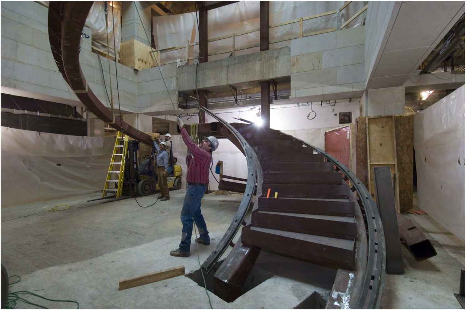
Clockwise from above: Workers position a curving steel beam into place in a stairwell atrium in Senate Expansion Space; a nearly completed corridor in House Expansion Space; along the face of the CVC's north entrance zone, a mason applies grout between the joint of two blocks of granite. The granite is quarried in Culpeper, Virginia, and is intended to match the perimeter walls around Capitol Square that were designed by Frederick Law Olmsted in 1874; a block of granite is lowered into place near one of two new elevator towers on the East Front Plaza. The elevators will bring people down approximately 18 feet from the Plaza to the CVC entrance level.
